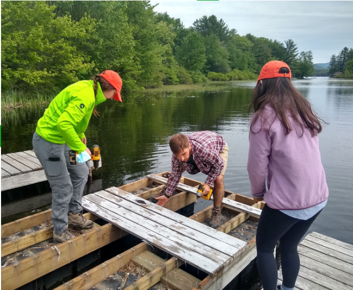
Above: LRCC Members repairing a dock.
